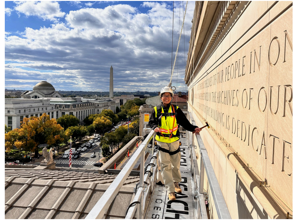
Constance Lai, FAIA, surveying the National Archives limestone facade from a swing stage, with two of her other projects in the background, the Smithsonian's National Museum of Natural History and the Washington Monument.
